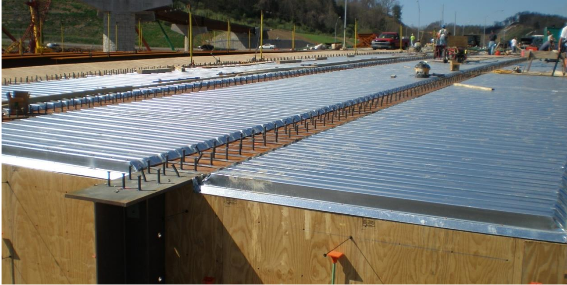
Figure 5 Photo showing permanent steel stay-in-place deck formwork installed on a steel plate I-girder bridge.
